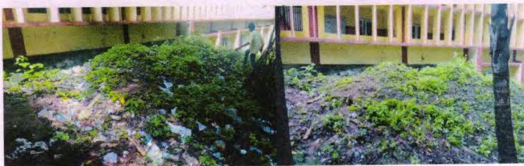
Before and After Cleaning
